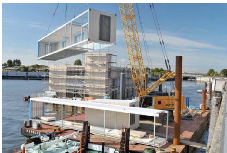
Figure 4. Modular construction, IBA Dock. (Source: http://www.archdaily.com/288198/iba-dock-architech/ , 2013.9)
