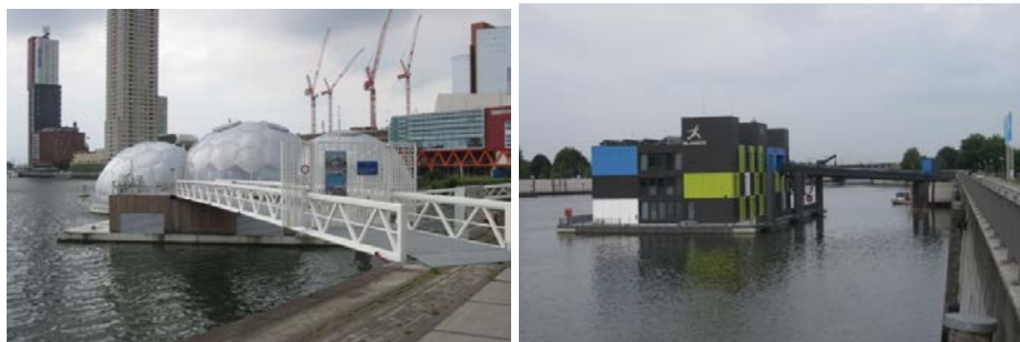
Figure 1 & 2. Floating Pavilion & IBA Dock
