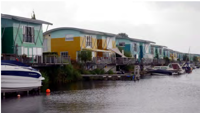
Figure 10. Overview of Floating Homes in DoudenKust
