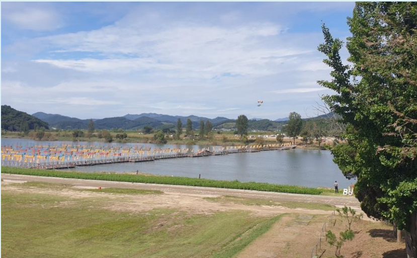
Temporary Floating Bridge for Festival Period
